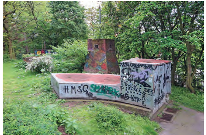
Graffitied entrance stairs and ventilation shaft of the Berliner Tor shelter. A second entrance can just be seen in the left middle distance.
